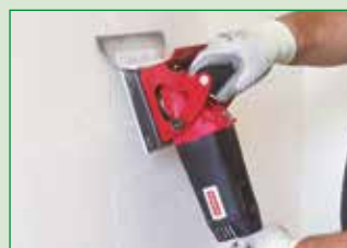
Application to the wall
