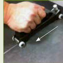
Arriving on the other wall, return the groover and start again from the skirting for finishing.
