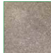
Concrete floors after
