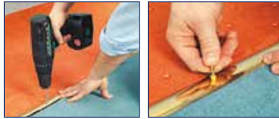
Drilling for Ø 3.5 mm raised countersunk head screws.
