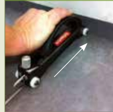
Arriving on the other wall, return the groover and start again from the skirting for finishing.
