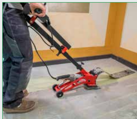
Push continuously but not roughly. (Do not use the machine as a scraper). Keep the blade at a 30° angle.
