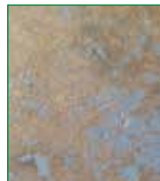
Concrete floors before
