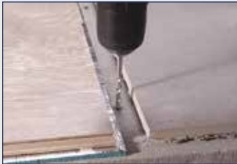
1- Before laying the floor-covering, draw a line and drill the desired number of holes (5/m) using a Ø 6 mm drill bit.
