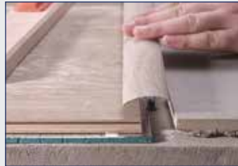
3- With the floor-covering installed, position the plugs opposite the holes.
