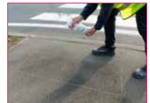
Application of activator
