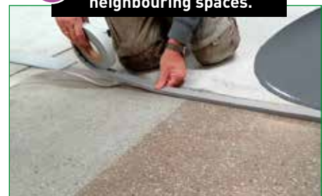
Delimitation of workspace Adhesive strips for adherence to the floor
