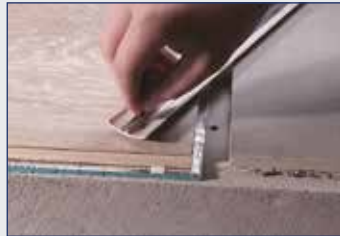
2- Insert the corresponding number of plugs into the profile and slide them into place.
