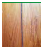
Vitrified wood floor before
